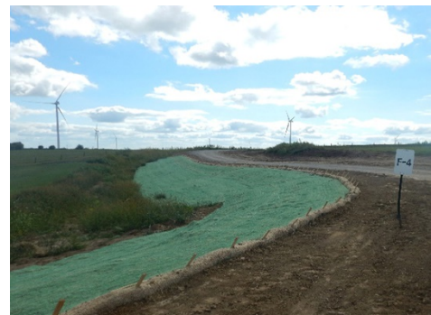
Figure 1 Hydroseeding slopes is an effective erosion control BMP.
