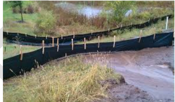
Figure 2 Silt fence should be installed along open soil perimeters.
