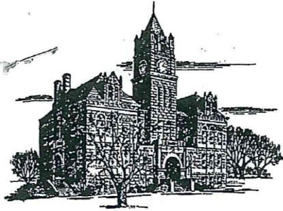
MARION COUNTY COURTHOUSE
